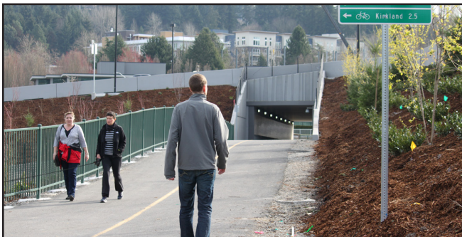
Pedestrians and bicyclists enjoy the new SR 520 regional shared-use path now open from Bellevue to Lake Washington.
