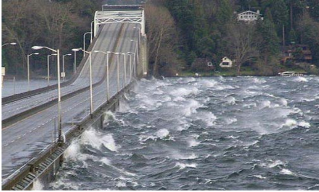
Waves batter the south side of the old, 1960s-era floating bridge during a February 2006 storm.
